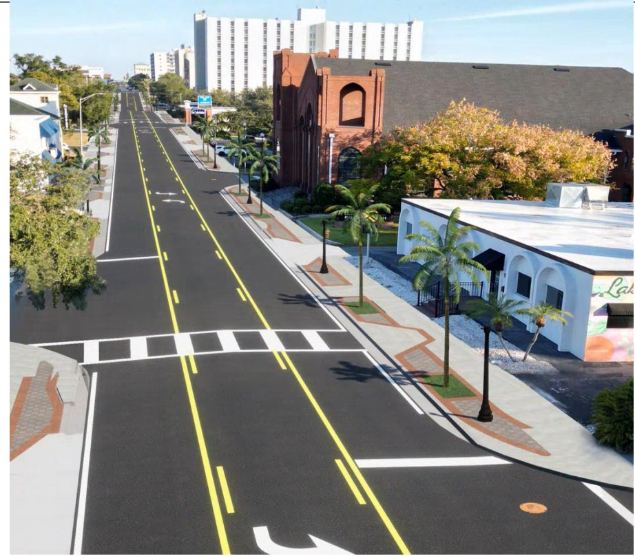
Looking northbound at Hilcrest Street
