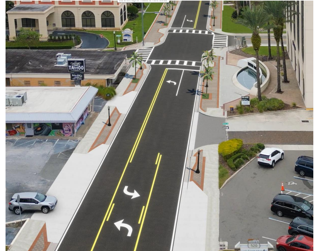
Looking northbound at Walnut Street
