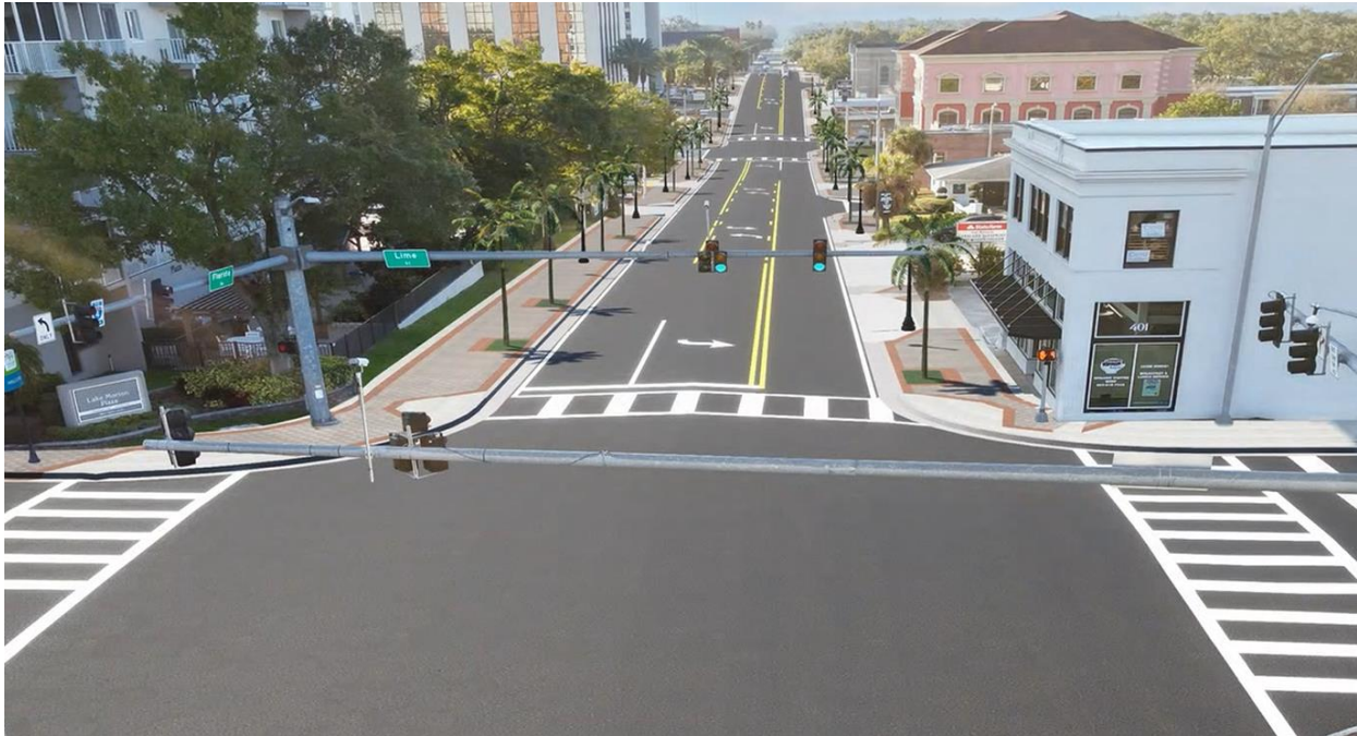
Looking southbound down SR 37 from Lime Street
